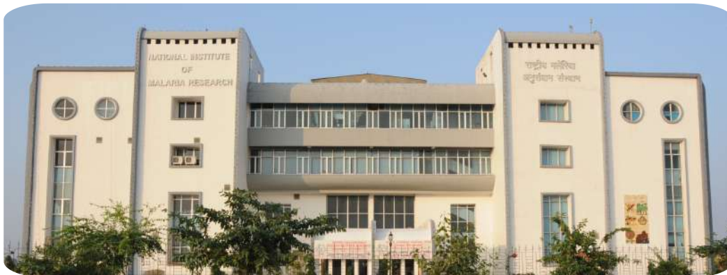
ICMR-NIMR building was established in 2005.
